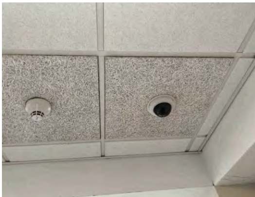
Item #: 1,036,568 Uniformat Number:C2050 Desc: Mismatched ACT - Fourth floor corridor
