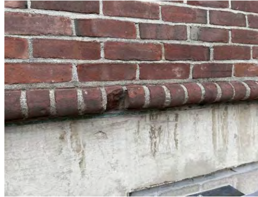
Item #: 1,032,678 Uniformat Number:B2010 Desc: Damaged brick - East elevation
