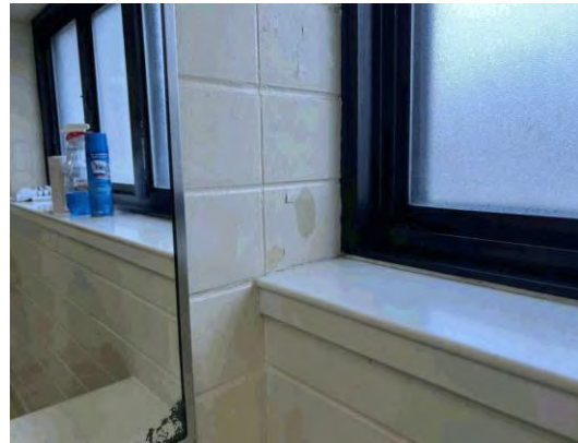
Item #: 1,036,669 Uniformat Number:C2010 Desc: Peeling paint - Bathroom 326
