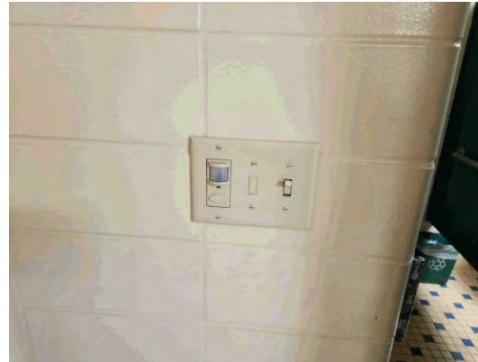
Item #: 1,036,190 Uniformat Number:D5040 Desc: Typical wall switch and occupancy sensor
