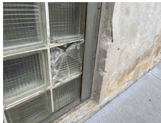
Item #: 1,032,693 Uniformat Number: B2020 Desc: Broken glass block - East elevation
