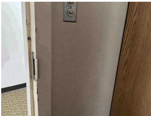
Item #: 1,036,666 Uniformat Number:C1030 Desc: Frame paint damage - Room 408
