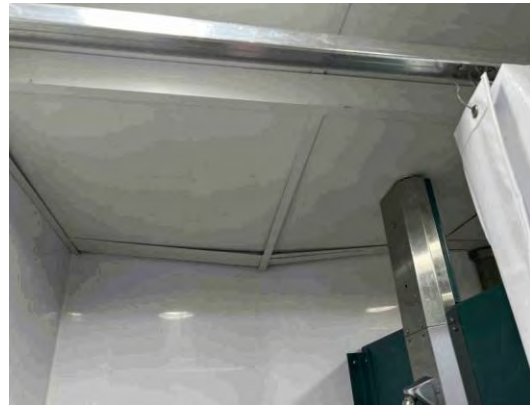
Item #: 1,036,568 Uniformat Number:C2050 Desc: Damaged ACT system - Bathroom 406
