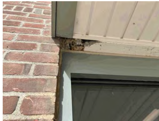
Item #: 1,032,678 Uniformat Number:B2010 Desc: Missing wood trim - South elevation
