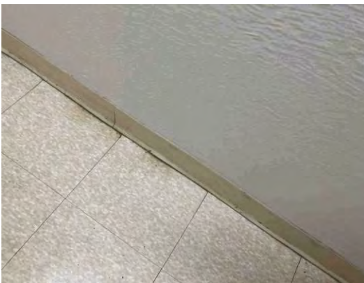
Item #: 1,036,669 Uniformat Number:C2010 Desc: Damaged wall base - Basement corridor
