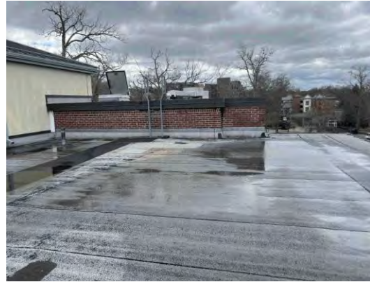
Item #: 1,036,555 Uniformat Number:B3010 Desc: Ponding
