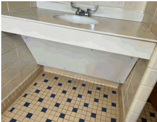
Item #: 1,036,601 Uniformat Number:C1090 Desc: Deteriorated sealant - Bathroom 406
