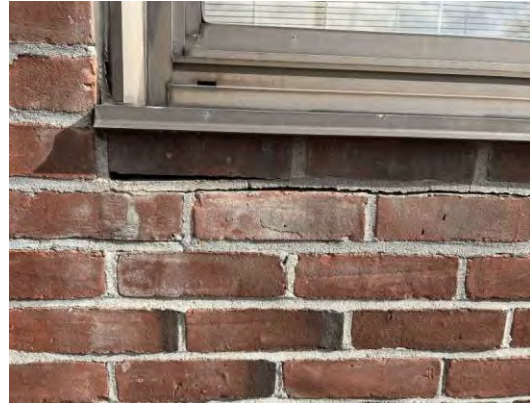
Item #: 1,032,678 Uniformat Number:B2010 Desc: Damaged mortar - West elevation
