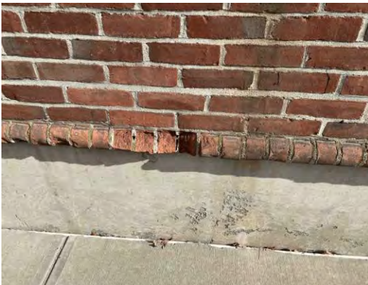
Item #: 1,032,678 Uniformat Number:B2010 Desc: Damaged brick - West elevation
