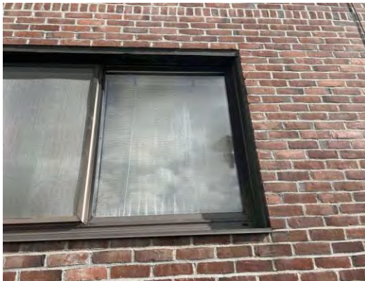
Item #: 1,032,693 Uniformat Number: B2020 Desc: Failed IGU - West elevation
