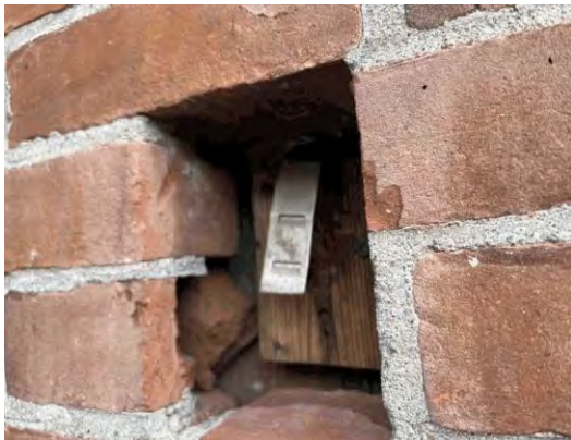
Item #: 1,032,678 Uniformat Number: B2010 Desc: Missing brick - West elevation
