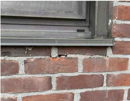
Item #: 1,032,678 Uniformat Number:B2010 Desc: Damaged mortar - East elevation
