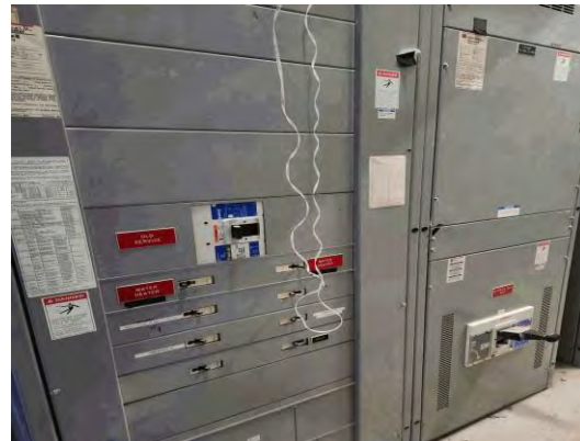
Item #: 1,036,187 Uniformat Number:D5020 Desc: Cutler-Hammer Switchboard
