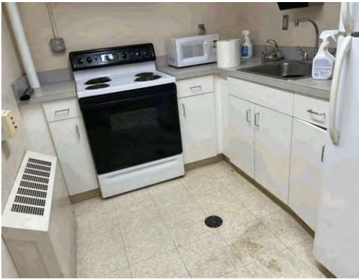
Item #: 1,036,594 Uniformat Number:C2030 Desc: Stained VCT - Kitchen 320
