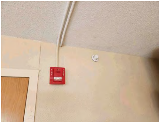
Item #: 1,036,185 Uniformat Number:D7050 Desc: A/V Alarm Notification Device
