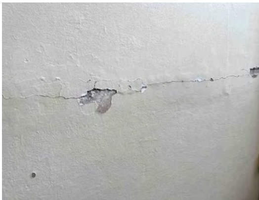
Item #: 1,036,674 Uniformat Number:A1010 Desc: Spalled concrete
