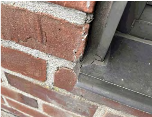
Item #: 1,032,678 Uniformat Number:B2010 Desc: Deteriorated sealant - East elevation
