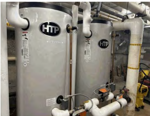
Item #: 1,036,865 Uniformat Number:D2010 Desc: Steam water heaters
