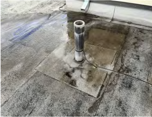
Item #: 1,036,555 Uniformat Number:B3010 Desc: Ponding
