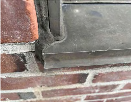
Item #: 1,032,678 Uniformat Number:B2010 Desc: Deteriorated sealant - West elevation
