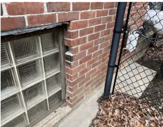
Item #: 1,032,678 Uniformat Number:B2010 Desc: Broken brick - East elevation
