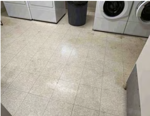
Item #: 1,036,594 Uniformat Number:C2030 Desc: Stained VCT - Laundry 004
