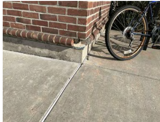
Item #: 1,032,678 Uniformat Number:B2010 Desc: Missing brick - Southwest elevation
