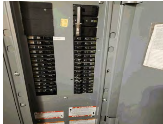
Item #: 1,036,186 Uniformat Number:D5020 Desc: Typical Panel with no arc flash hazard warning label
