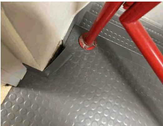
Item #: 1,036,669 Uniformat Number:C2010 Desc: Damaged wall base - Basement stair
