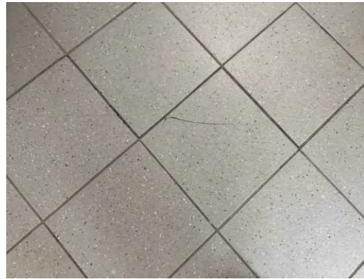
Item #: 1,036,594 Uniformat Number:C2030 Desc: Cracked tile - Second floor lobby
