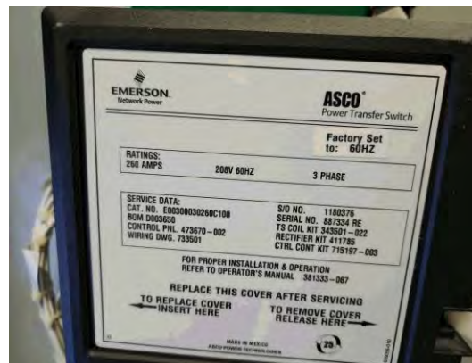
Item #: 1,036,188 Uniformat Number:D5010 Desc: ATS- E nameplate
