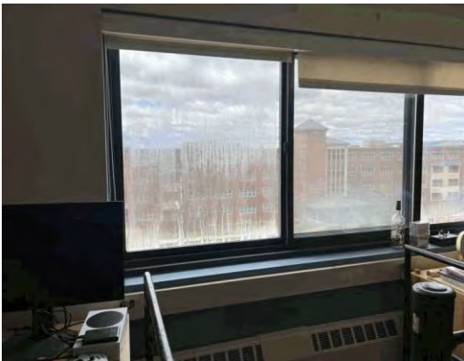
Item #: 1,032,693 Uniformat Number:B2020 Desc: Failed IGU - Room 325
