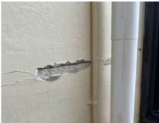
Item #: 1,036,674 Uniformat Number:A1010 Desc: Spalled concrete
