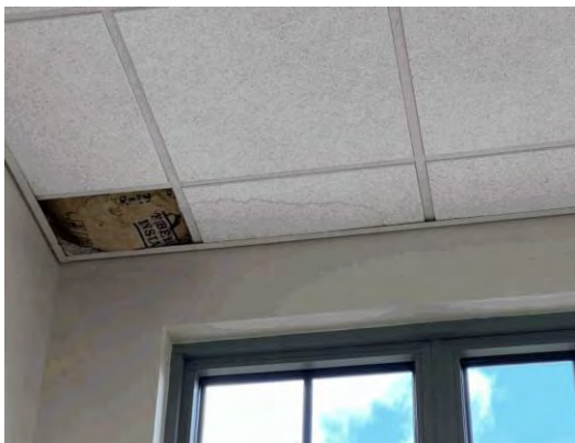
Item #: 1,036,568 Uniformat Number:C2050 Desc: Missing tile - Fourth floor lobby
