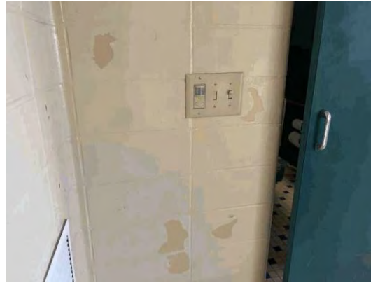
Item #: 1,036,669 Uniformat Number:C2010 Desc: Peeling paint - Bathroom 326
