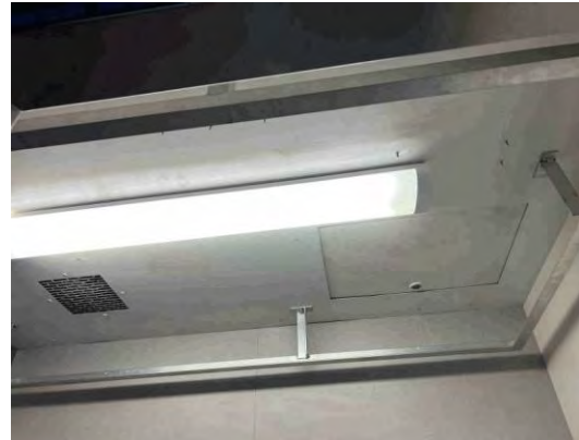
Item #: 1,036,563 Uniformat Number:D1010 Desc: Missing ceiling
