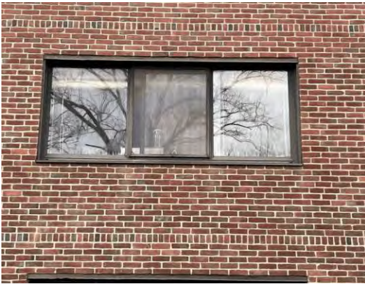
Item #: 1,032,693 Uniformat Number:B2020 Desc: Failed IGU - East elevation
