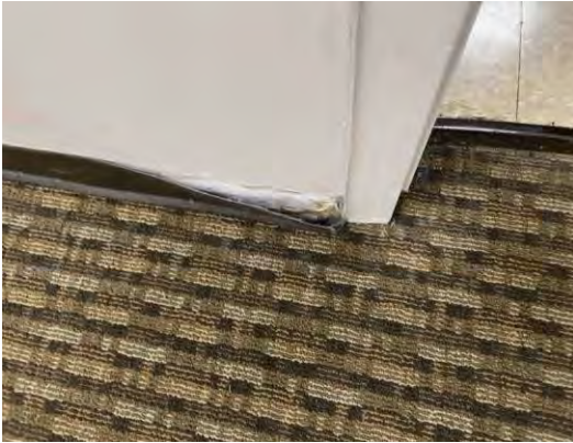
Item #: 1,036,669 Uniformat Number:C2010 Desc: Damaged wall base - Third floor corridor
