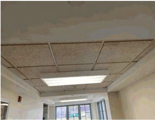
Item #: 1,036,568 Uniformat Number:C2050 Desc: Stained ACT - Third floor corridor
