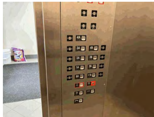
Item #: 1,036,563 Uniformat Number:D1010 Desc: Cab controls
